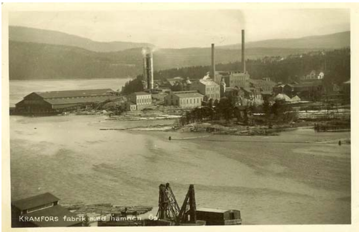
The Kramfors pulp and paper factory in 1934. Although the dumping of many contaminants is now regulated, there are banks of waste that were created before the legislation was introduced that are now threatening the ecosystem as they are dispersed. Photo from http://www.famqus.se/Gudmund/SagFab-Kramfors.htm
